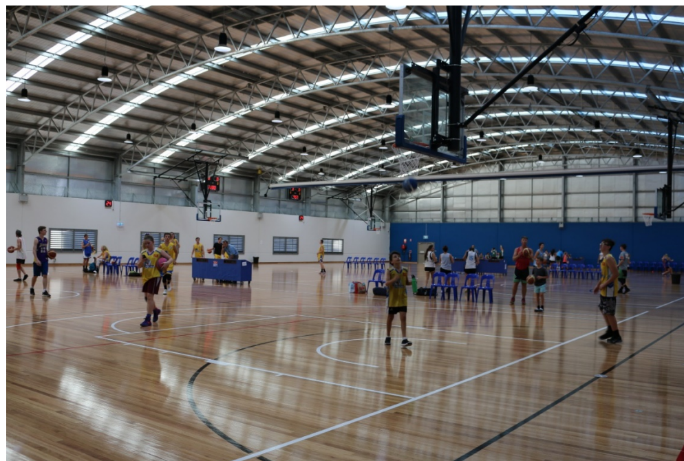
Port Macquarie Indoor Stadium upgrade
