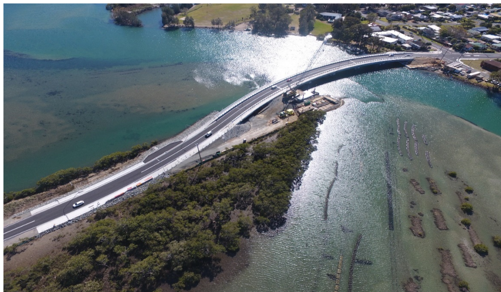
Stingray Creek Bridge upgrade
