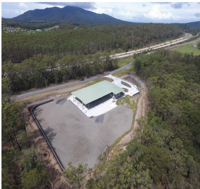
Kew Waste Transfer station
