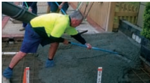
Right: Footpath works Far right: Rainbow Beach Playground
