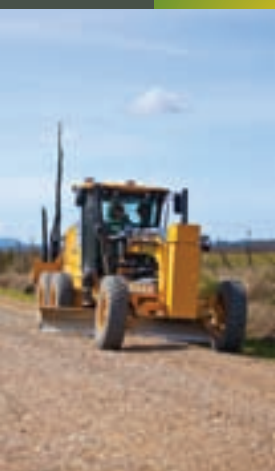
Above: Road grading
