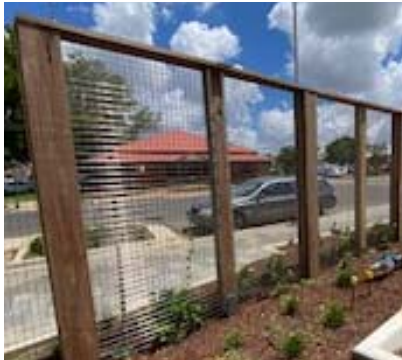
GREEN WALL - RECYCLED TIMBER & SS
