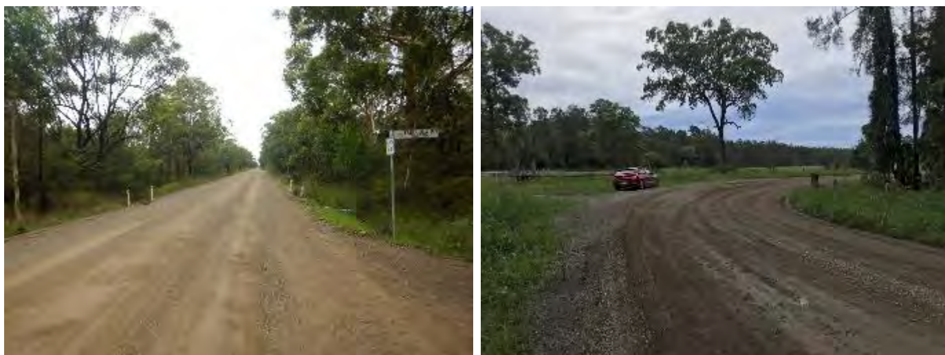
Figure 4.4 Typical existing delineation condition of Maria River Road on straights and on curves
