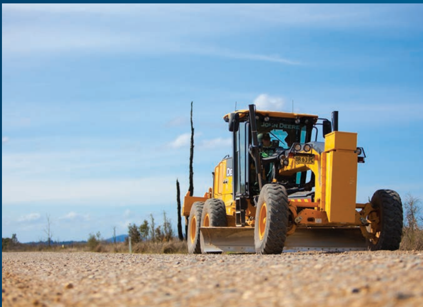
Unsealed Road grading
