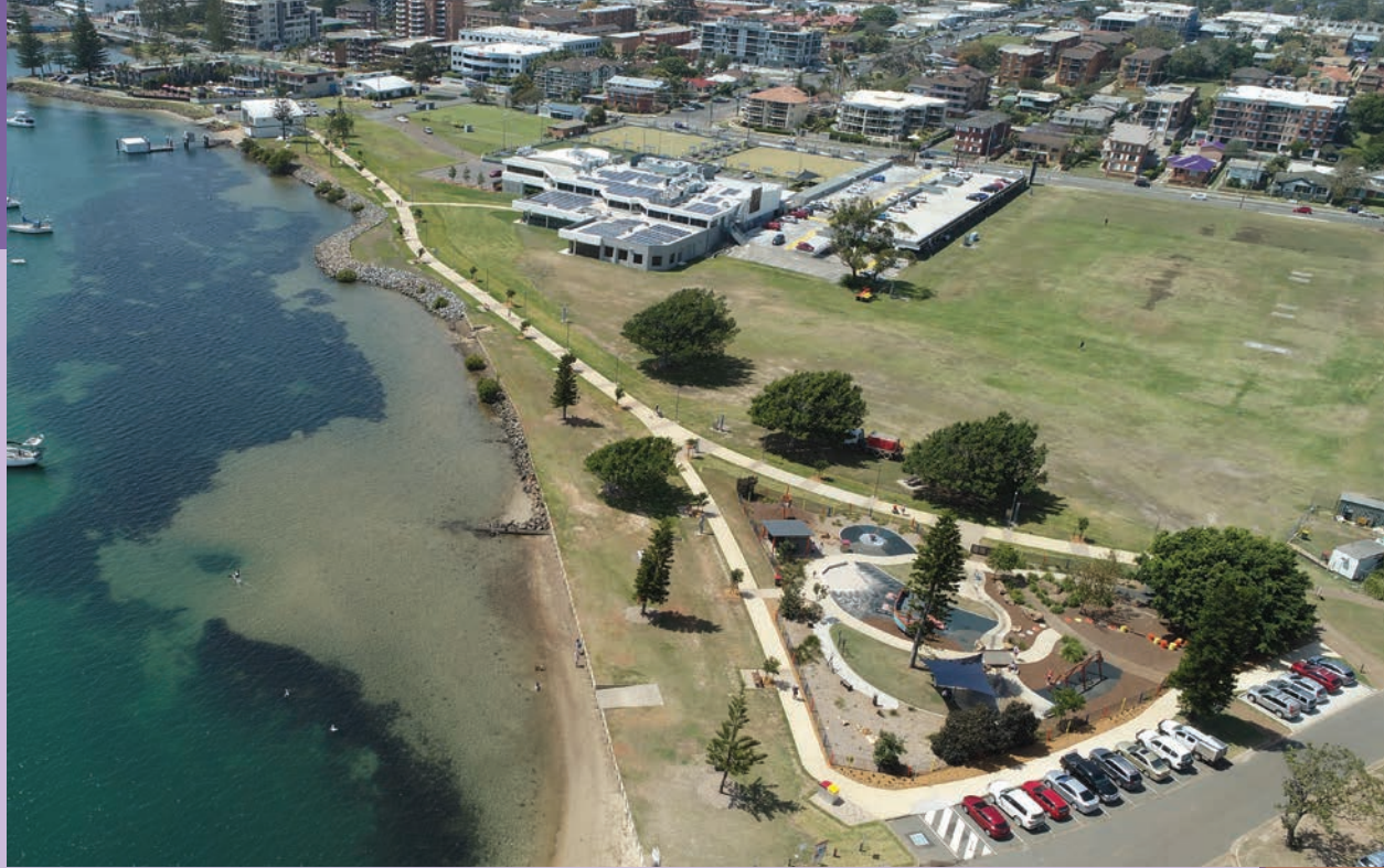
Coastal Walk, Westport Park Segment
