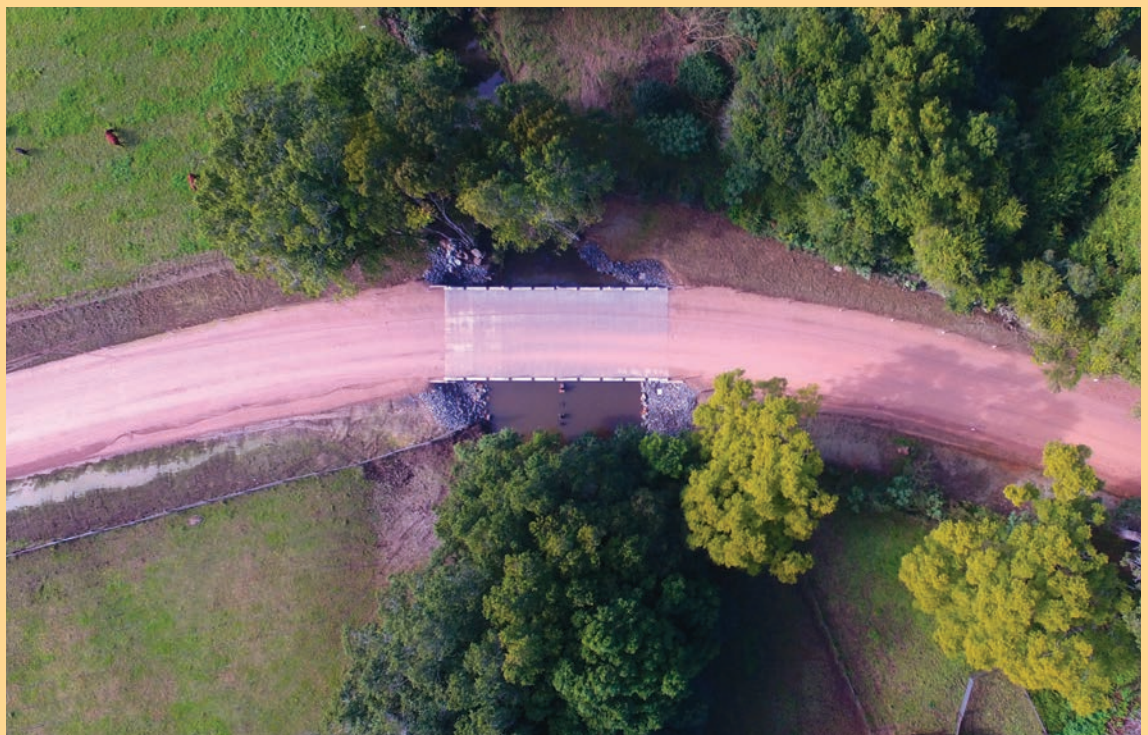
O'Neill's Bridge, Batar Creek Road
