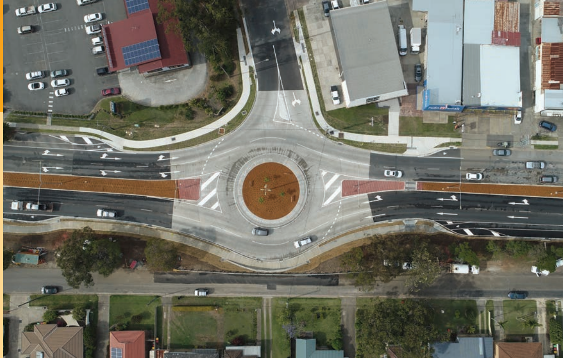
Newport Island Roundabout
