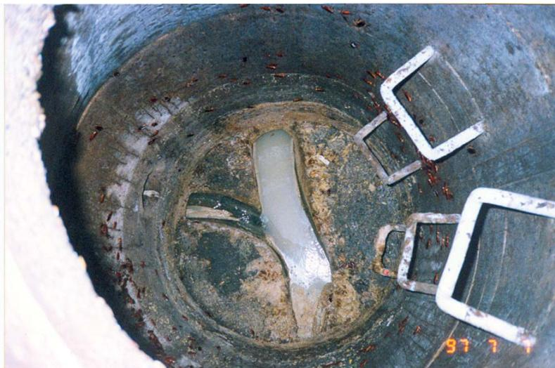
*Fat build-up in manhole – almost completely blocking outlet*
