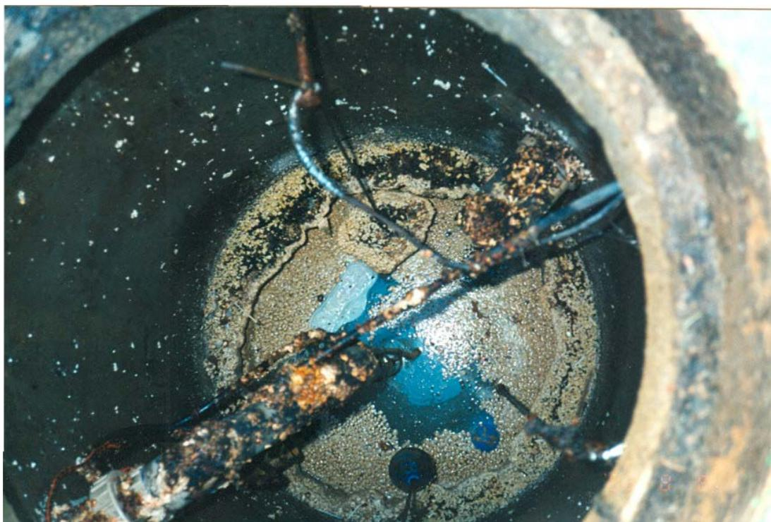
Grease & oil in private sewer pump station showing build-up of grease & damage to pumps
