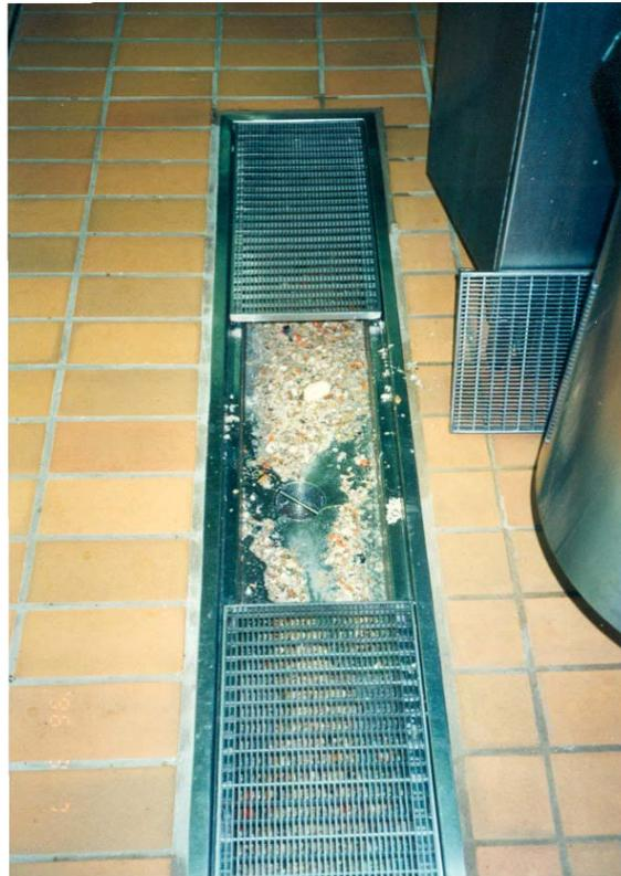
*Back-up into kitchen graded drain due to sewer choke caused by grease and oil.*
