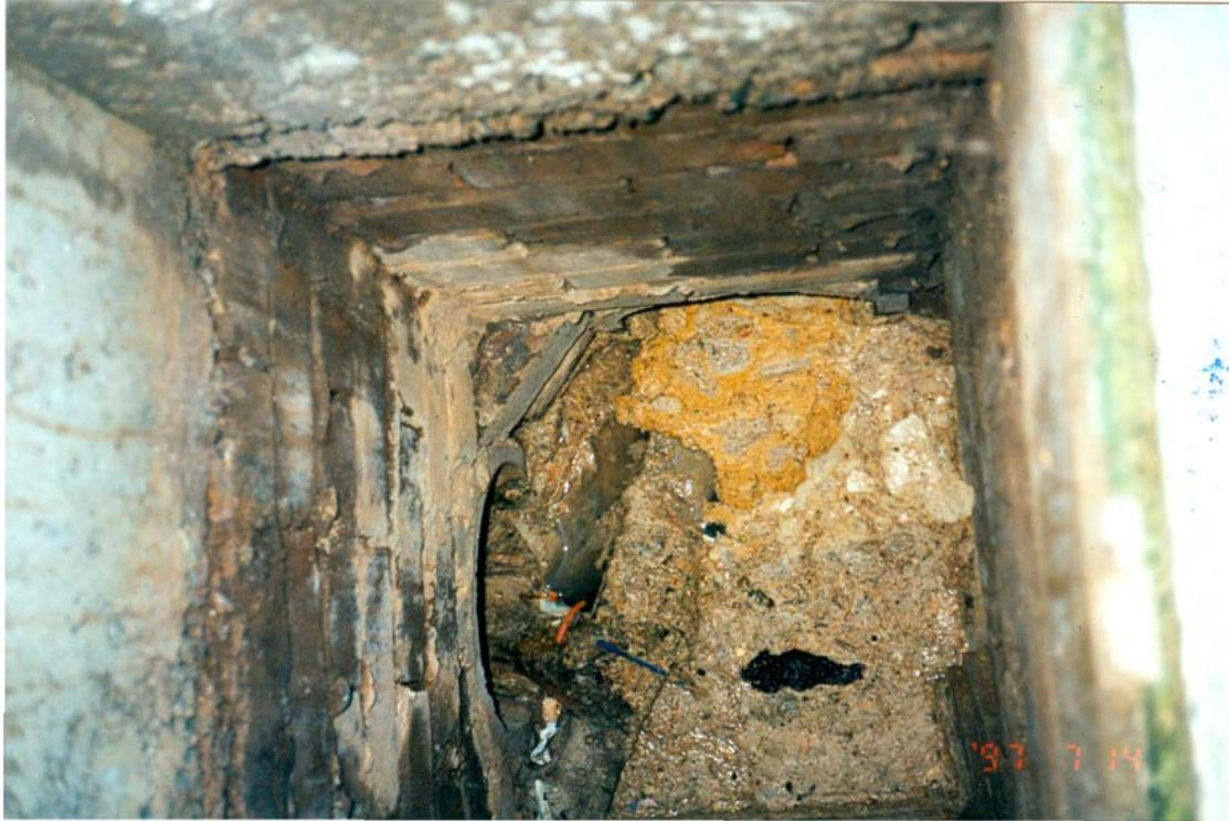
*Grease & oil entering stormwater pit from uncontrolled trade waste*
