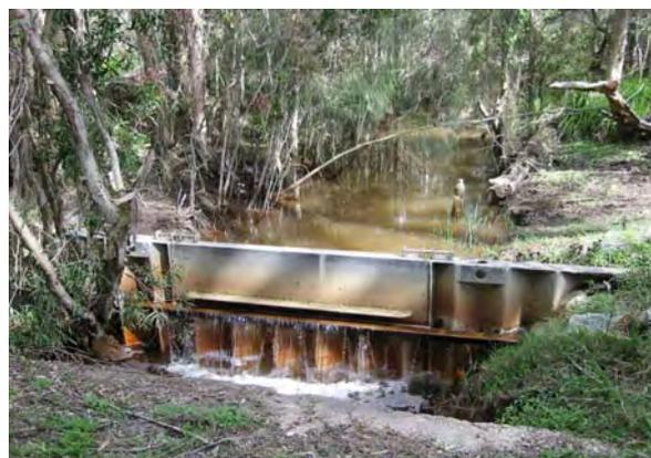
Weir in artificial drain restoring the hydrology of a 300-heactre wetland, and reducing acid discharge into the Maria River
